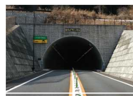
Number of Road Tunnels 596 (as of Mar 31, 2019)
